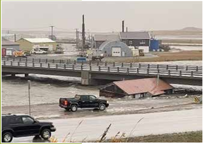
A house is stuck under the Snake River bridge in Nome. Credit: Emily Schwing / Alaska Department of Transportation
